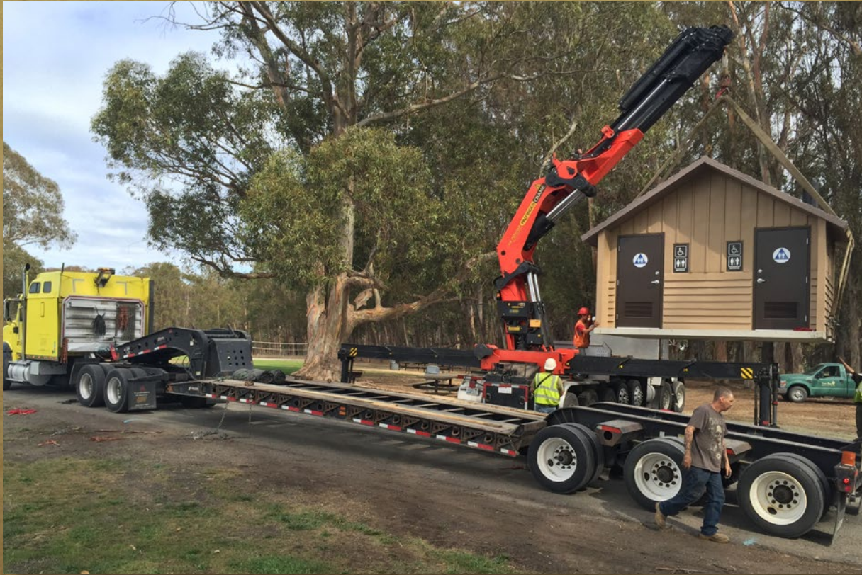
Point Pinole Restroom Installation
